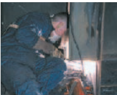
Figure 8. MMA welding with OK 73.68.
