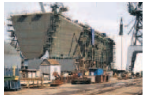
Figure 11. LPG tank under construction.
