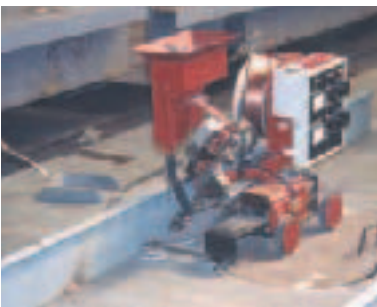
Figure 7. Single-sided SAW welding with OK Autrod 12.32/OK Flux 10.62.
