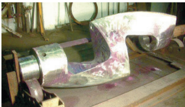
Fig. 2. Repair welded mixer blade ready for profiling by grinding.
