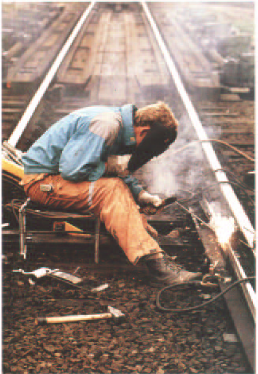
Figure 1. By weld surfacing of track components such as crossings, switch blades and so on, length of service can be substantially prolonged at a lower cost than to replace the worn component with a new one.
