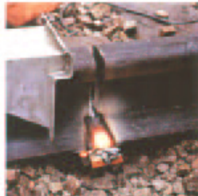
Figure 8. Welding of the foot using electrode OK 74.78.
