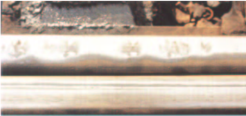
Figure 4. "Squats" due to rolling contact fatigue.
