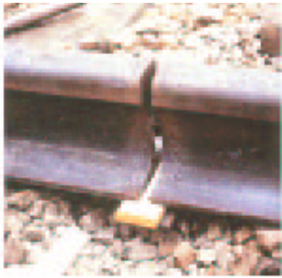
Figure 7. Mounting of backing, OK Backing 21.21.
