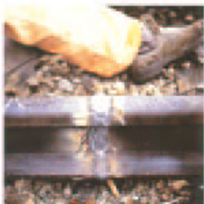
Figure 10. Complete weld before grinding.
